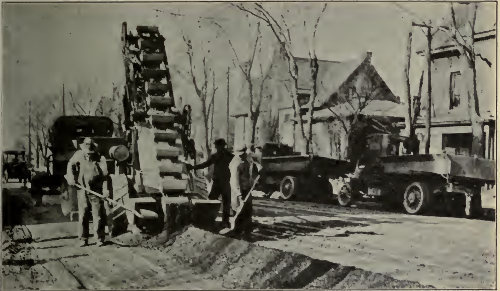
REMOVING EXCESS MATERIAL AFTER SCARIFYING AND RESHAPING MACADAM STREET IN DENVER PRIOR TO APPLICATION OF SHEET ASPHALT TOP
